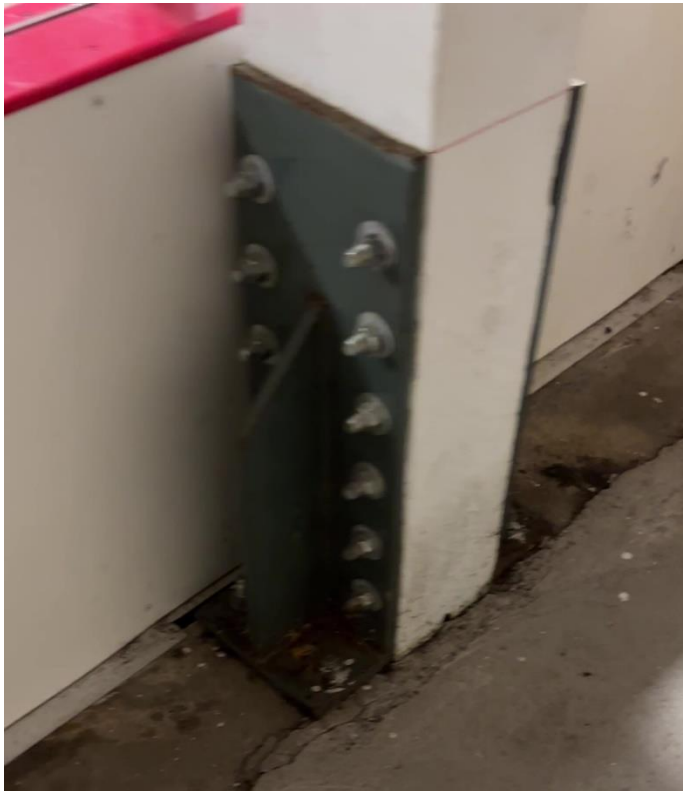
Photo: Steel Bracket Reinforcing
